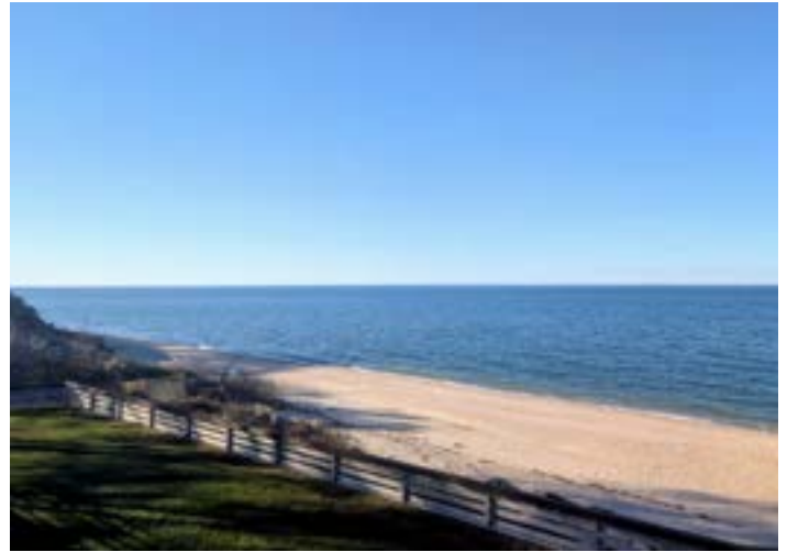
View of the Sound from Village Hall in Shoreham. The conceptual designs developed through this project will help improve stormwater management in the Village and ultimately water quality in Long Island Sound. Credit: Elizabeth Hornstein.
