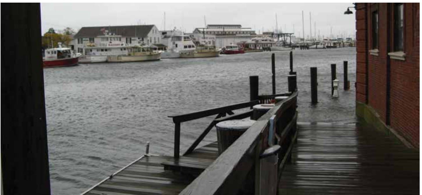
The Main Block building is one of several locations in downtown Mystic prone to flooding. Photo courtesy of Town of Groton
