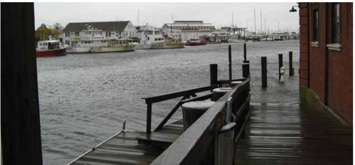
The Main Block building is one of several locations in downtown Mystic prone to flooding. Photo courtesy of Town of Groton
